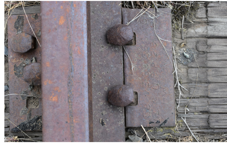
EXPOSED STEEL & WOOD
