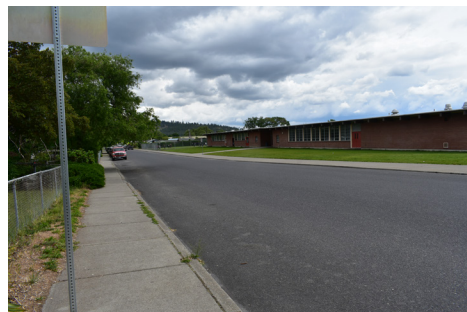
EXISTING SHAW MIDDLE SCHOOL
