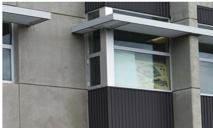
PRE-CAST CONCRETE & METAL SIDING
