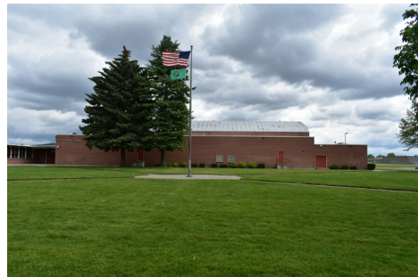
EXISTING SHAW GYMNASIUM WEST
