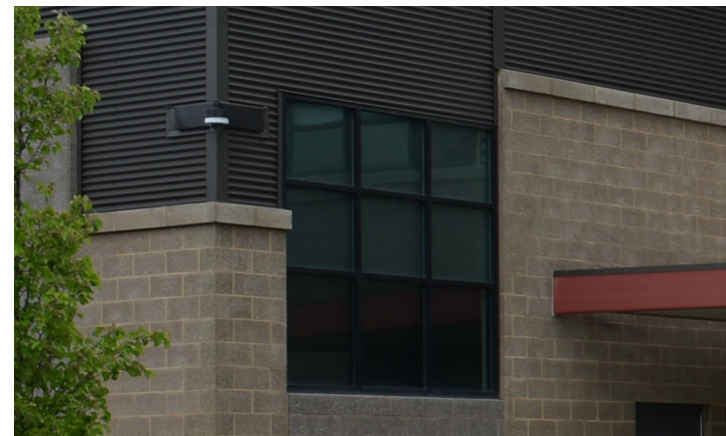
CONCRETE MASONRY UNIT & METAL SIDING
