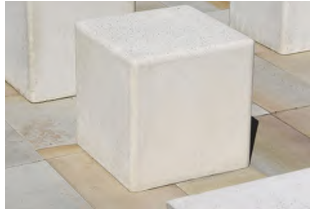
Cubic bollards provide seating and force protection.
