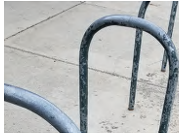
Painted metal fabrications need frequent maintenance.
