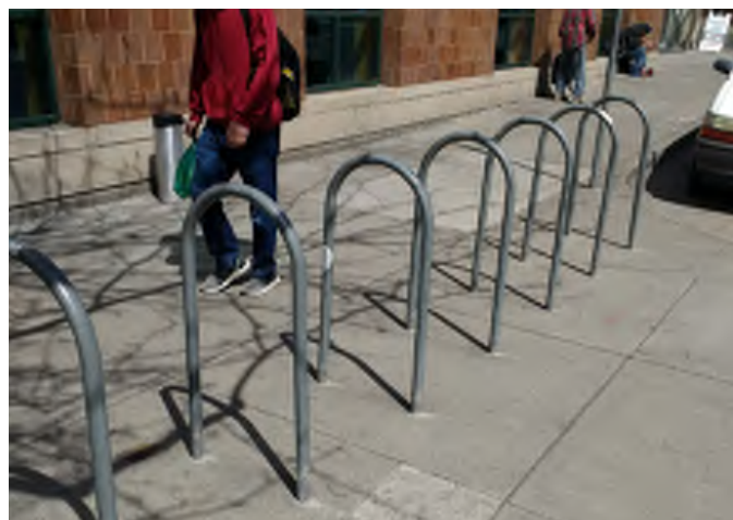
Painted metal fabrications need frequent maintenance.
