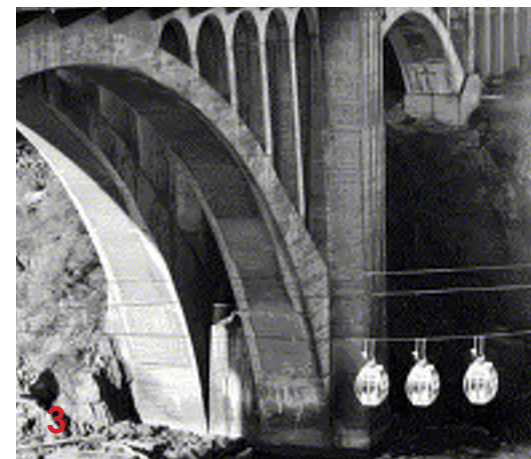
SPOKANE RIVER & MONROE BRIDGE
