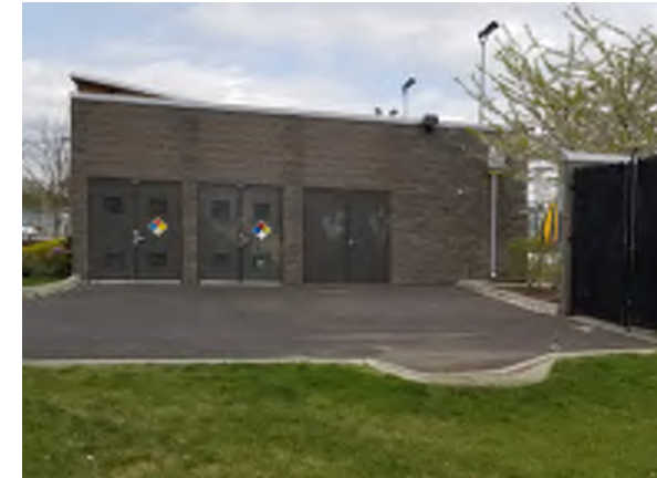
View of adjacent aquatic center service yard will need screening from entry plaza.
