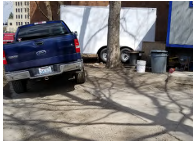
Construction activities have damaged existing tree roots and paving.
