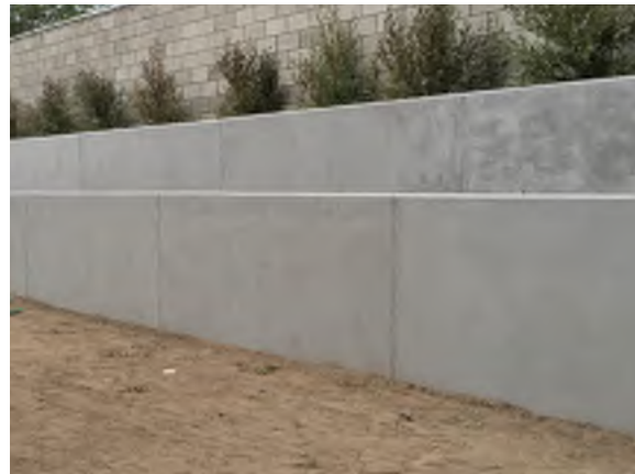
Smooth form cast-in-place concrete retaining walls are simple and timeless.
