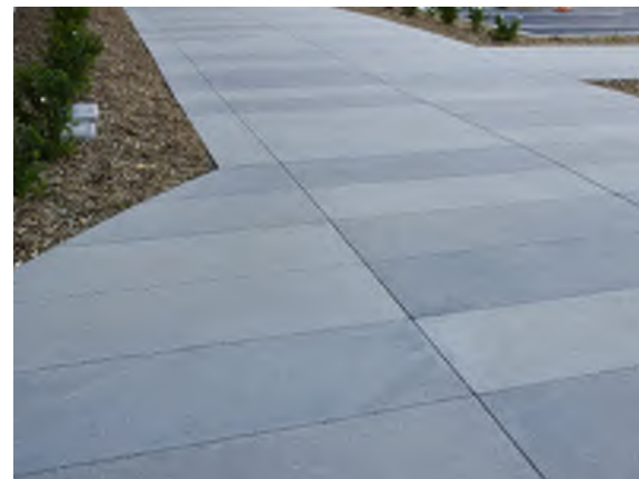
Integral color concrete plaza paving.
