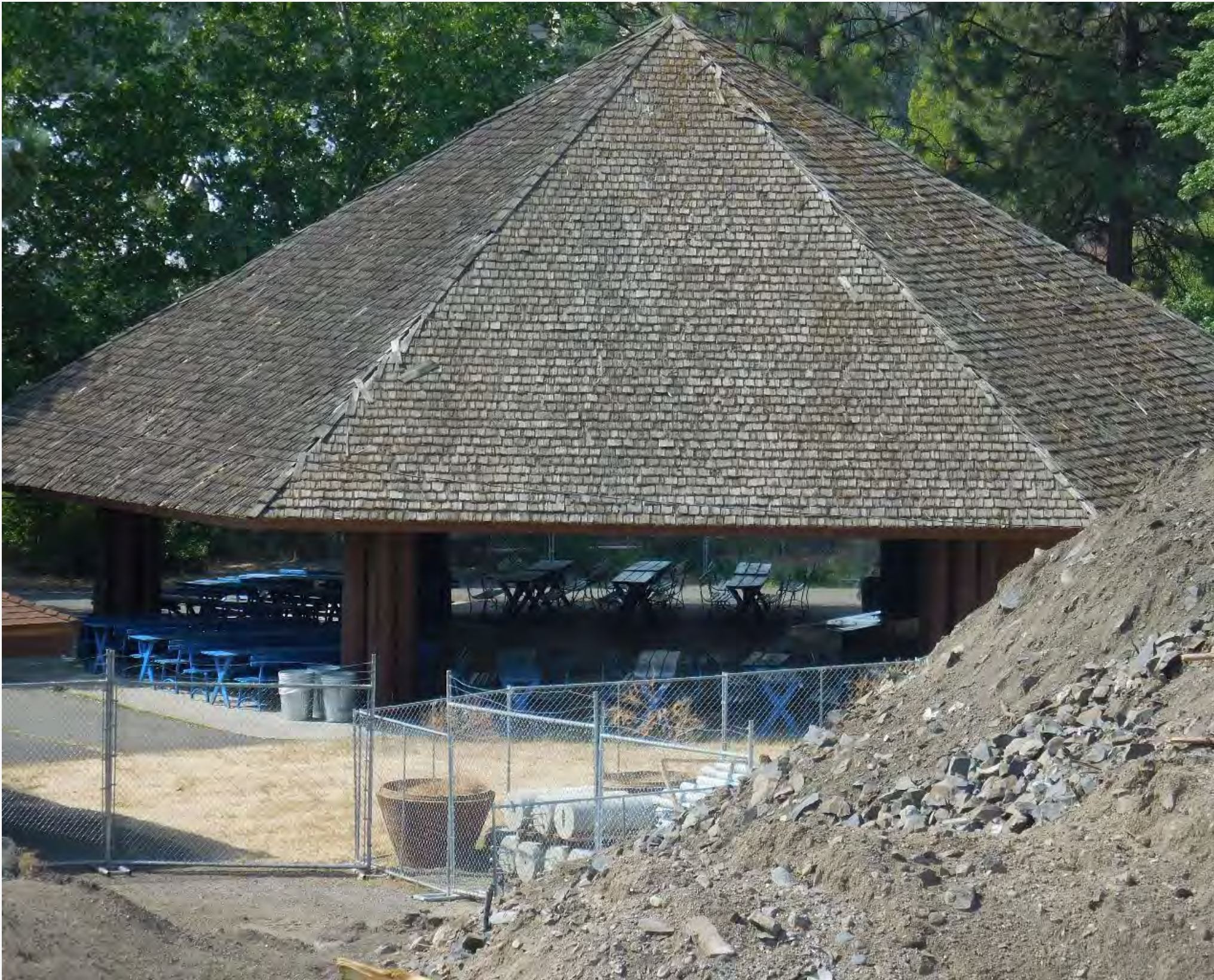
EXISTING PICNIC SHELTER TO REMAIN
