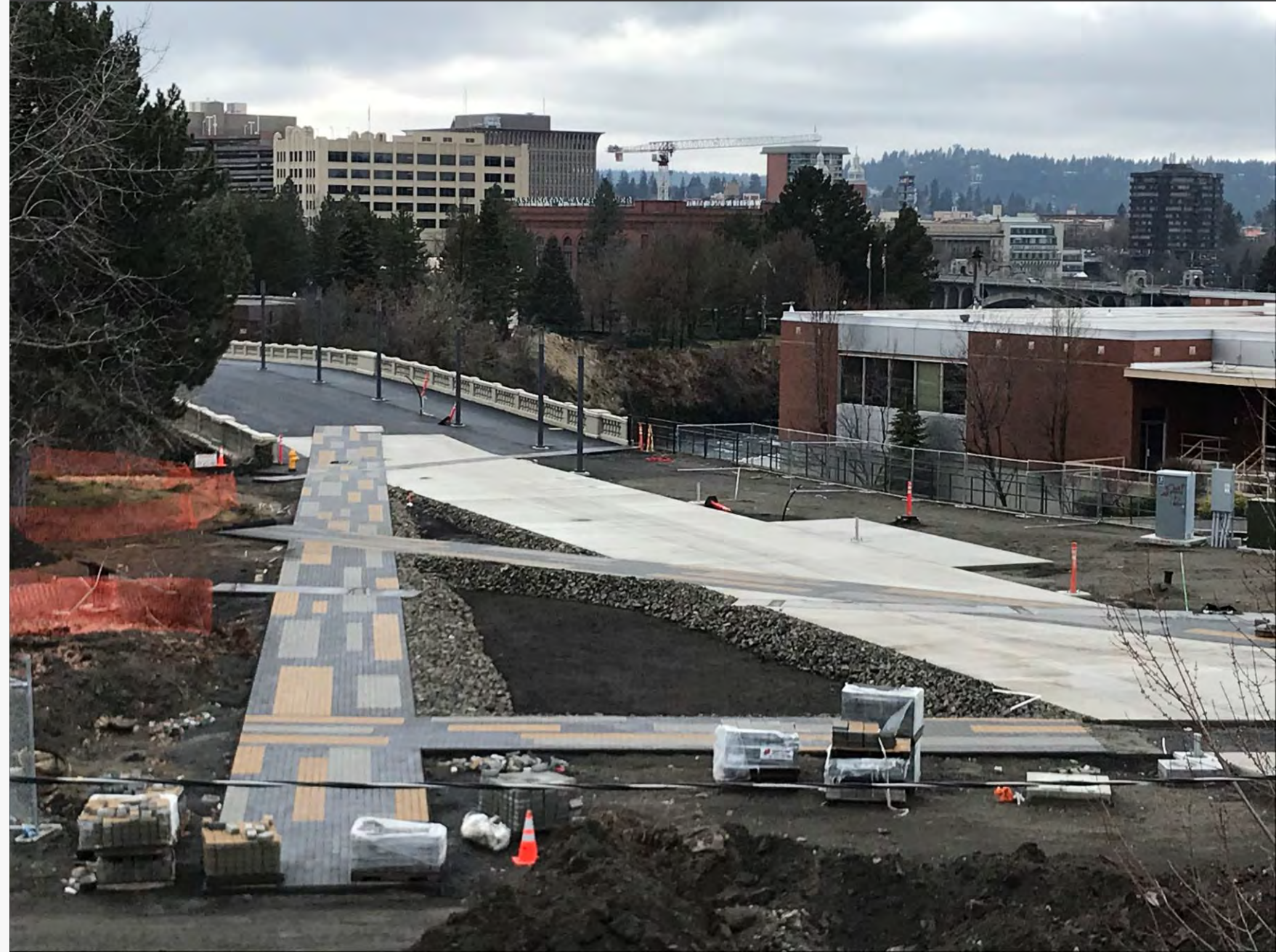
NORTH HOWARD PROMENADE CONSTRUCTION
