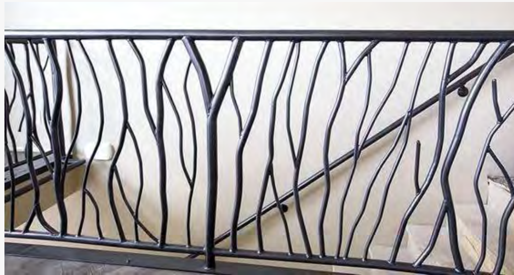
DECORATIVE RAILING AT PLAYGROUND
