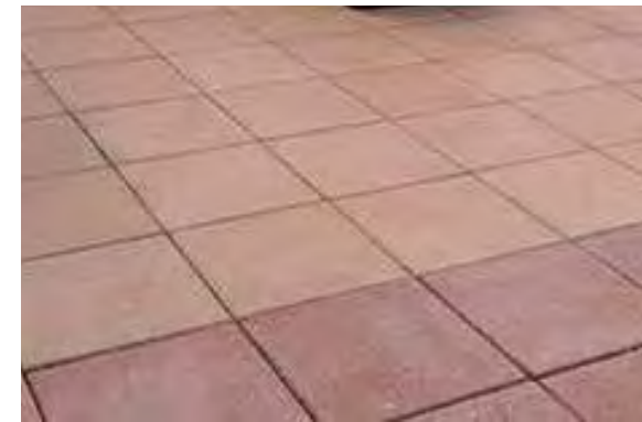
PEDESTAL PAVERS AT ROOF TERRACE
