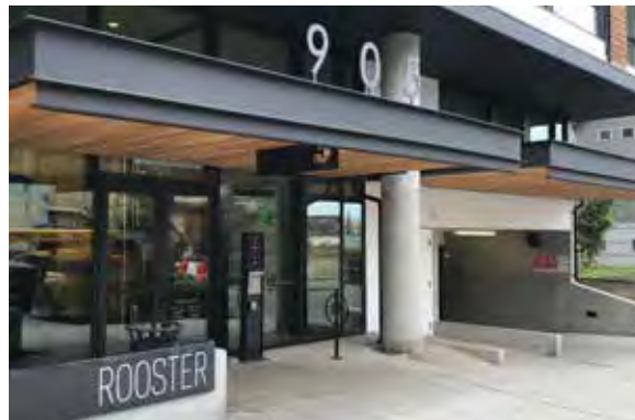
REAR ENTRY ADJACENT TO SERVICE
