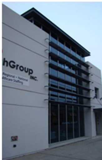
Portion of roof extended.
