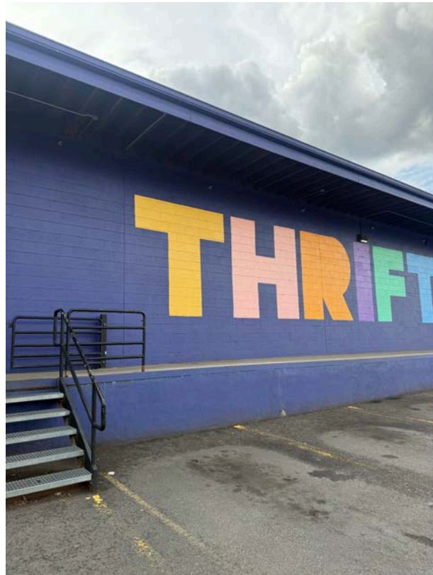
Figure 36: Picture showing large empty platform outside of Global Thrift.
