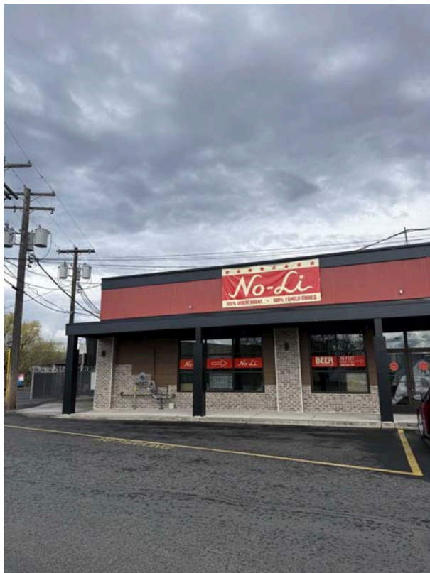
Figure 35: Picture emphasizing lack of infrastructure outside of NoLi Brewhouse.
