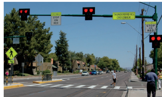
Example of a pedestrian hybrid beacon (top) and location options for Westview Ave. and Graves Rd. PHBs (right).
