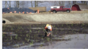
Constructed stormwater wetland during construction.
