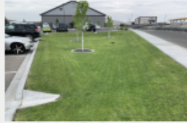
Bioswale BMP in Eastern Washington.
