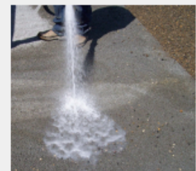
Runoff infiltrates through permeable pavement.
