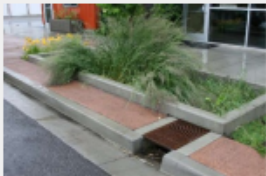
Bioretention cells are an example of LID BMPs.
