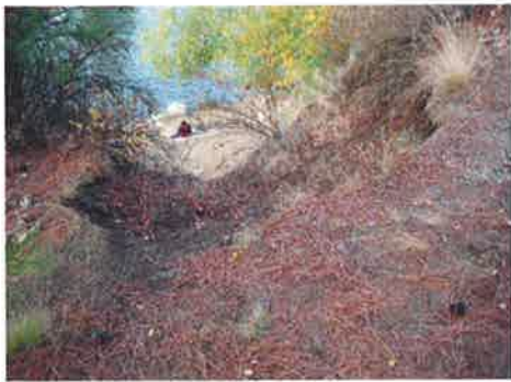
Eroded Pedestrian pathway from top.
