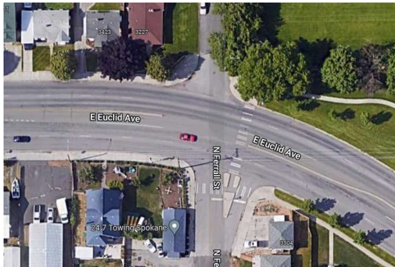
Euclid Avenue and Ferrall Street Intersection
