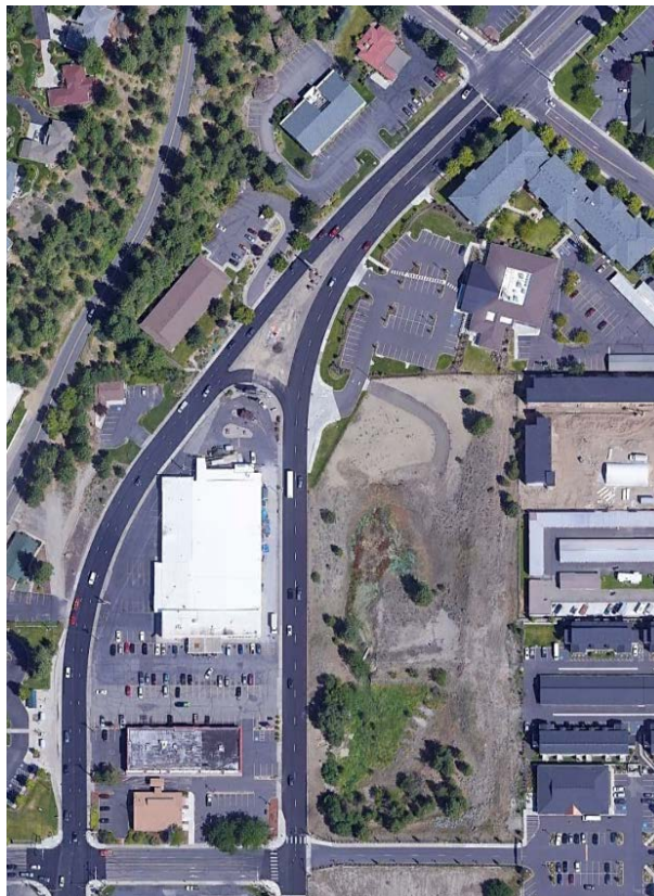
Maple Street and Ash Street at Country Homes Boulevard Intersection
