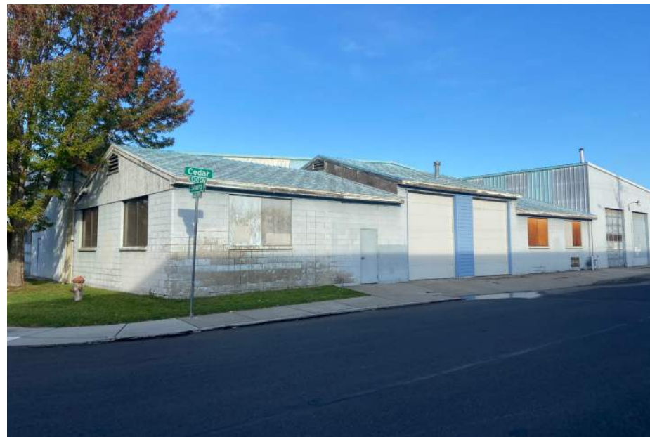
EXISTING BUILDING - EAST SIDE
